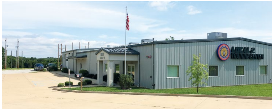
IBEW Local 2 Training Center.
